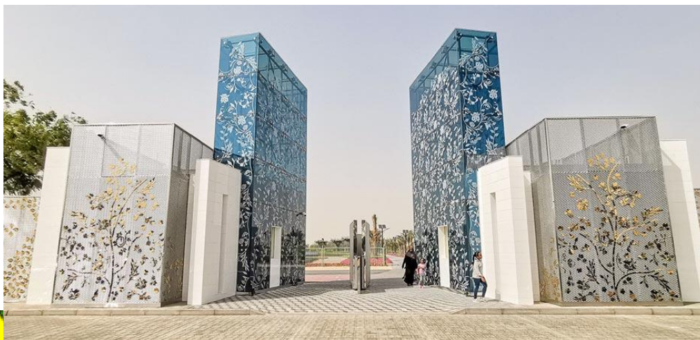
Gambar 9.8; Pintu masuk Quranic Garden menerapkan elemen sense of welcoming and safety
